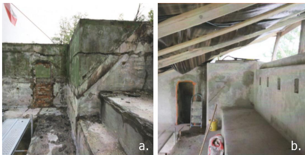
Fig. 5. The condition of the shooting gallery after the disassembly of the roof (a.) and during conservatory works (b.).
