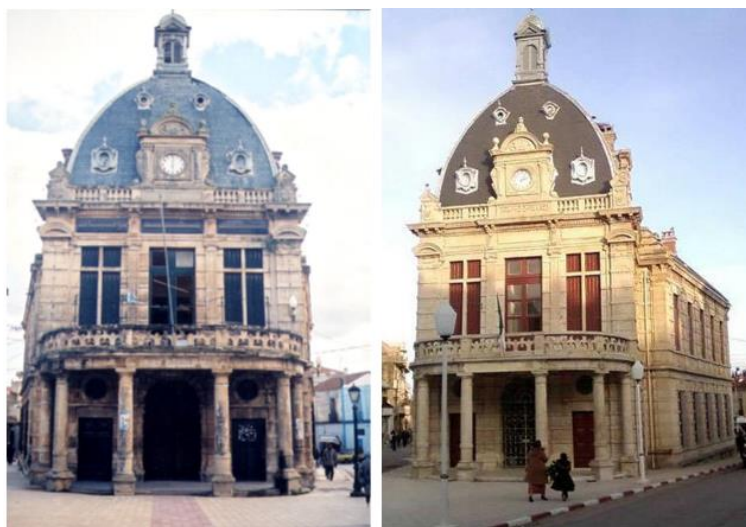
Fig. 2. City Hall before and after rehabilitation
